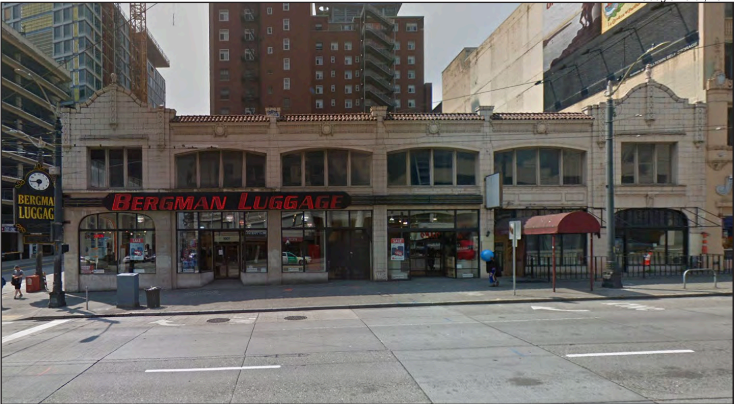
Figure 82 • Donohoe Garage (Now Bergman Luggage), 1901 Third Avenue, built 1921
