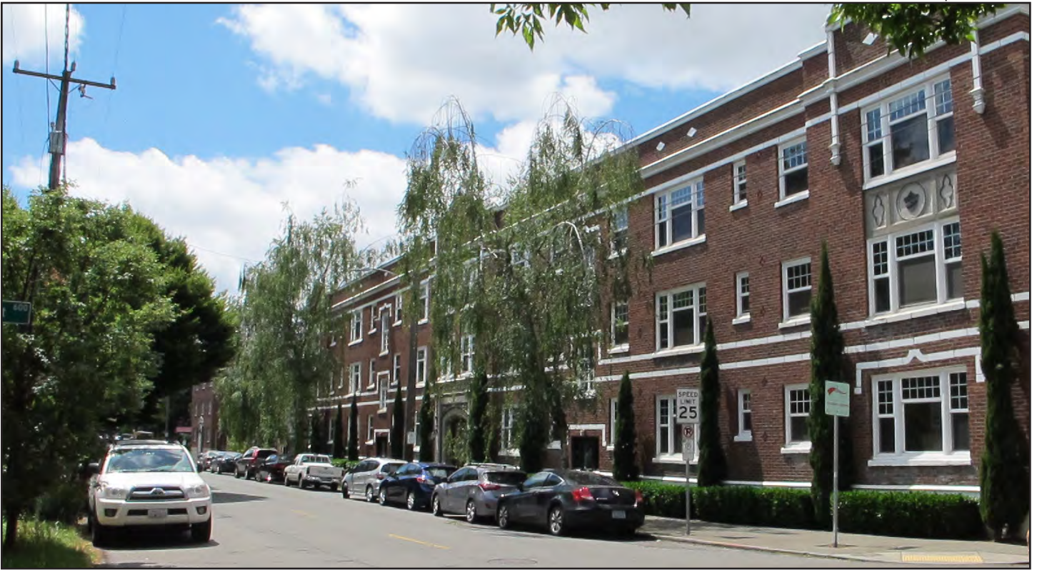
Figure 13 • 615 Bellevue Avenue E, eastern façade
