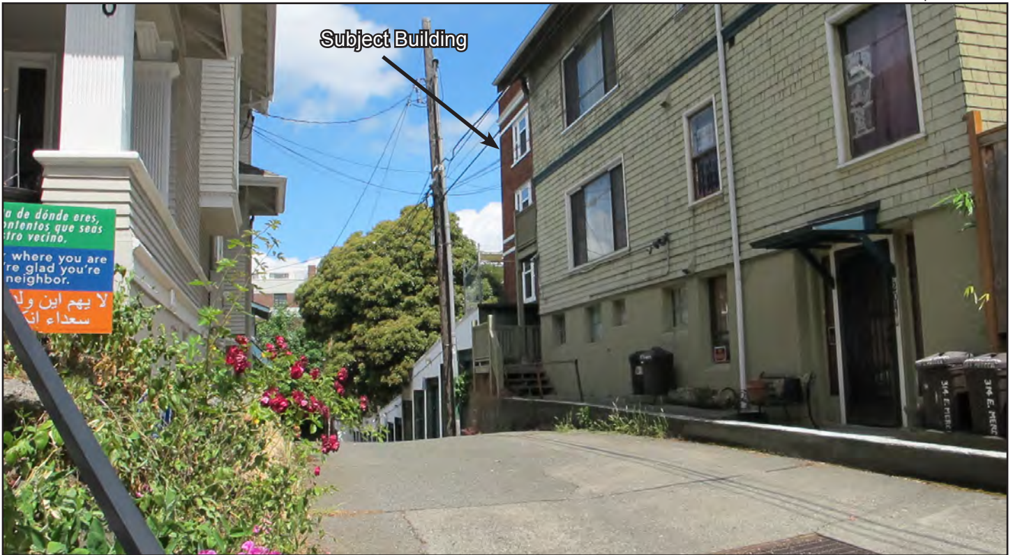
Figure 6 • View C - Viewing north on rear alley from E Mercer Street
