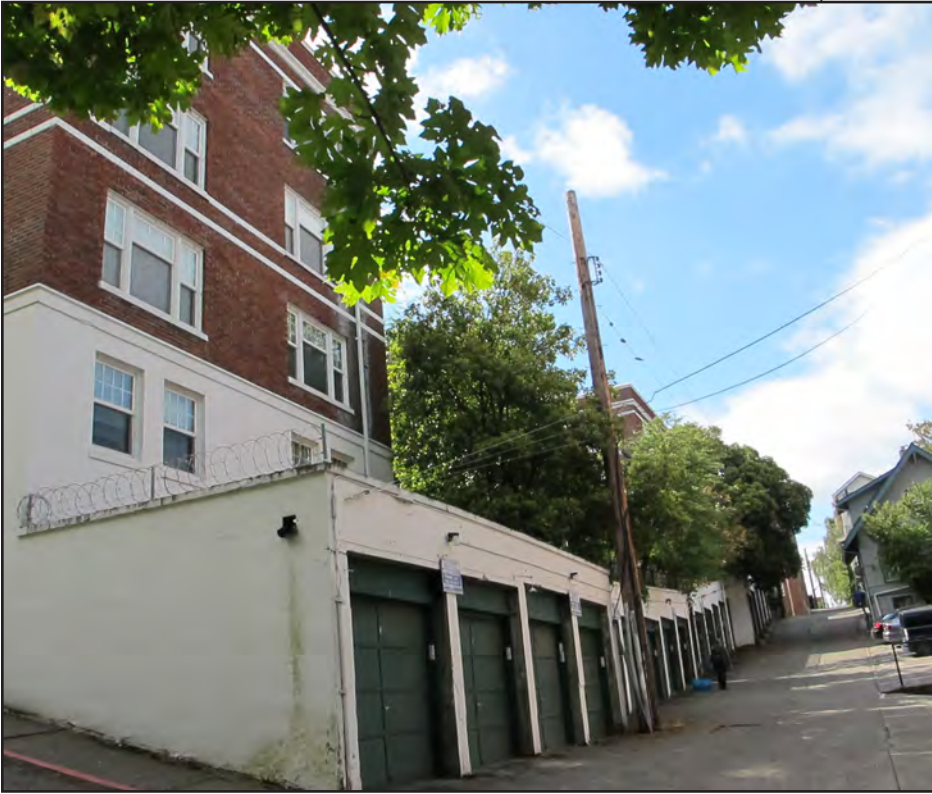
Figure 29 • Western façade, northern wing, alley looking south from E Roy Street
