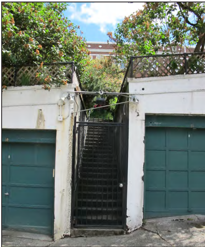
Figure 32 • Western façade, garden exit onto rear alleyway
