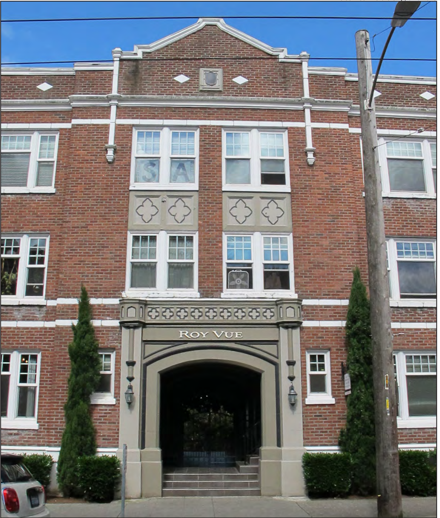
Figure 15 • Eastern façade, central porch and main entrance
