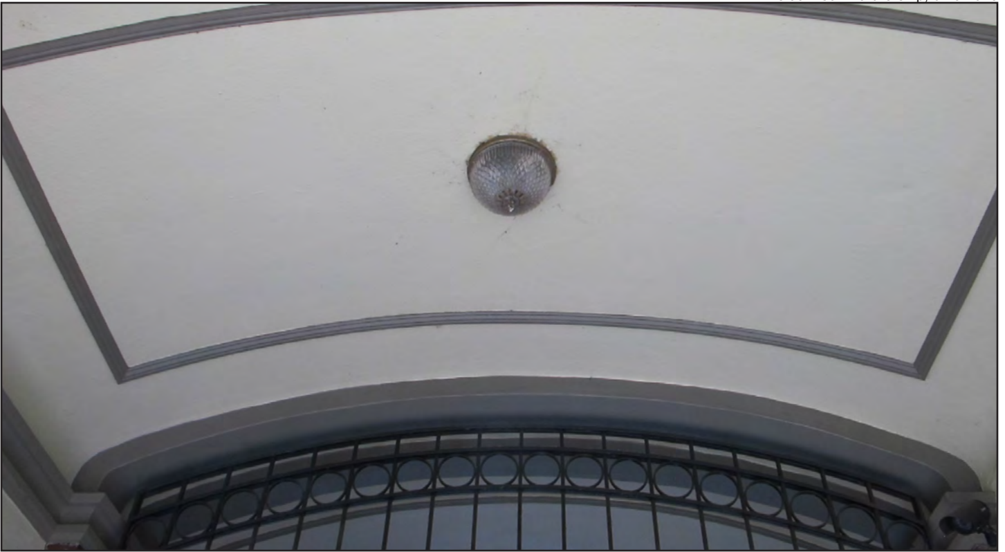
Figure 18 • Eastern façade, detail of main entry ceiling
