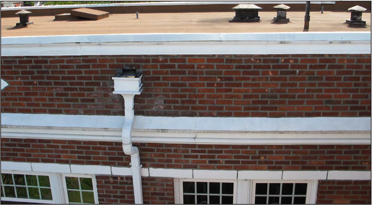
Figure 37 • Courtyard-east façade, roof detail
