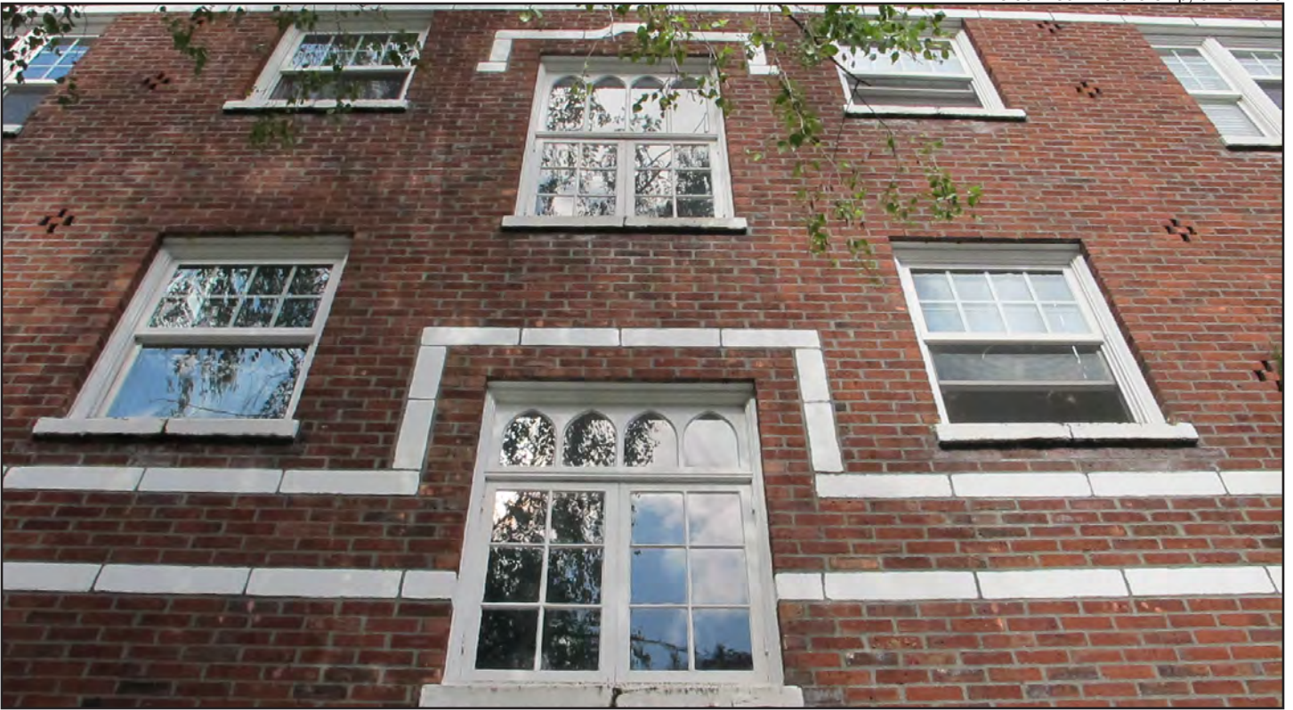
Figure 16 • Eastern façade, window detail
