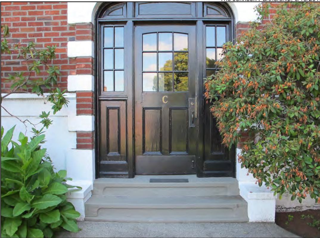
Figure 40 • Courtyard-east façade, example of courtyard primary entrance stairs
