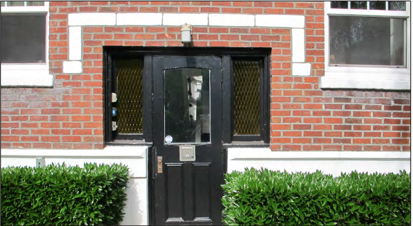
Figure 20 • Eastern façade, exterior secondary stairs with hood- or label mold
