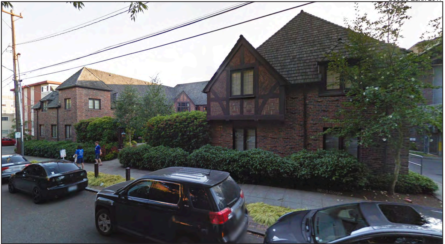
Figure 80 • Anhalt Harvard Avenue Apartments, Tudor, built 1929
