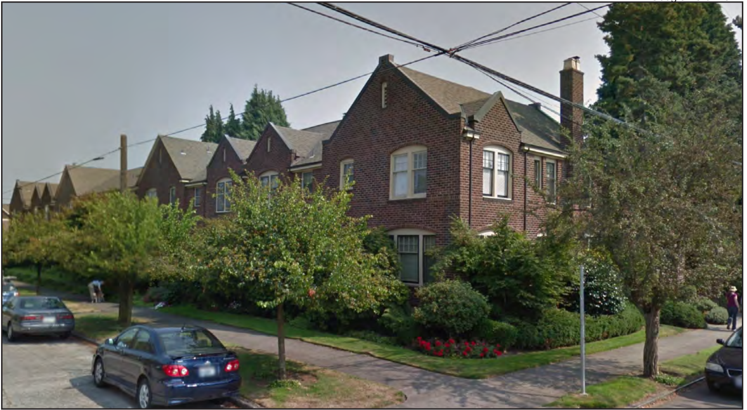
Figure 79 • Hawthorne Square in Fremont, Tudor, built 1924
