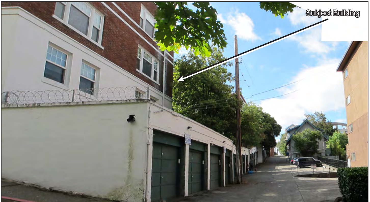
Figure 7 • View D - Viewing south on rear alley from E Roy Street
