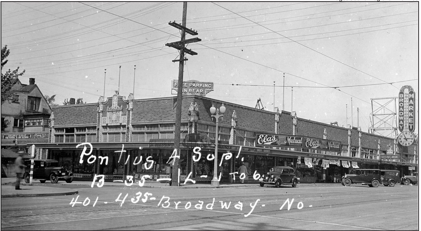
Figure 83 • Broadway Market (401 Broadway E) in 1937, built 1928
