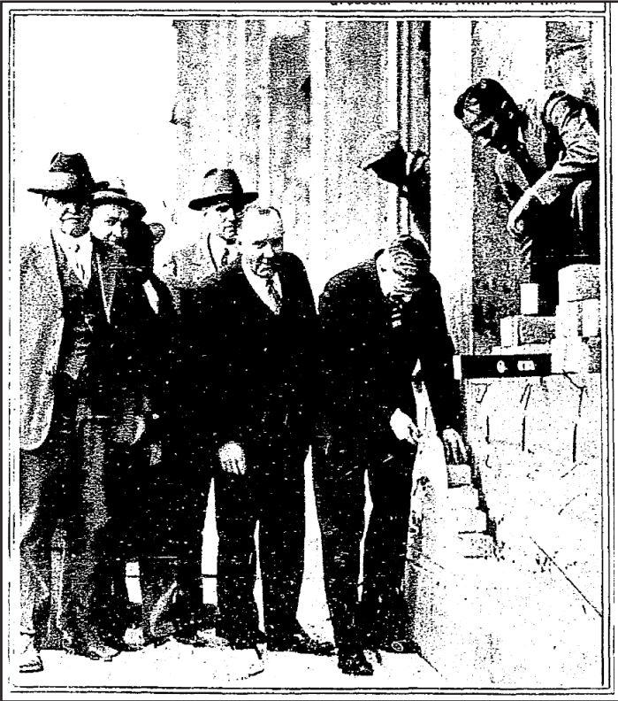
Figure 88 • County-City Building Addition, 1929, Hans Pederson (far left)
