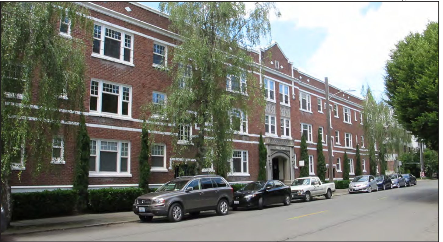
Figure 12 • 615 Bellevue Avenue E, eastern façade
