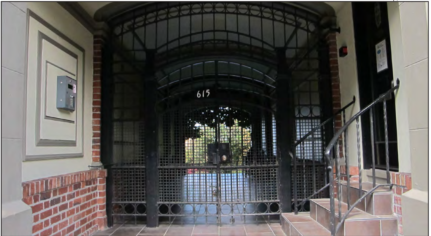
Figure 19 • Eastern façade, gated main entry
