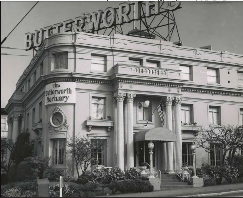
Figure 81 • Butterworth Mortuary, 300 E Pine Street, built 1922
