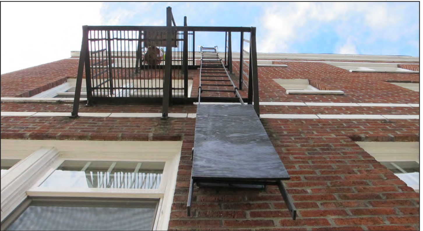
Figure 28 • Northern façade, fire escape
