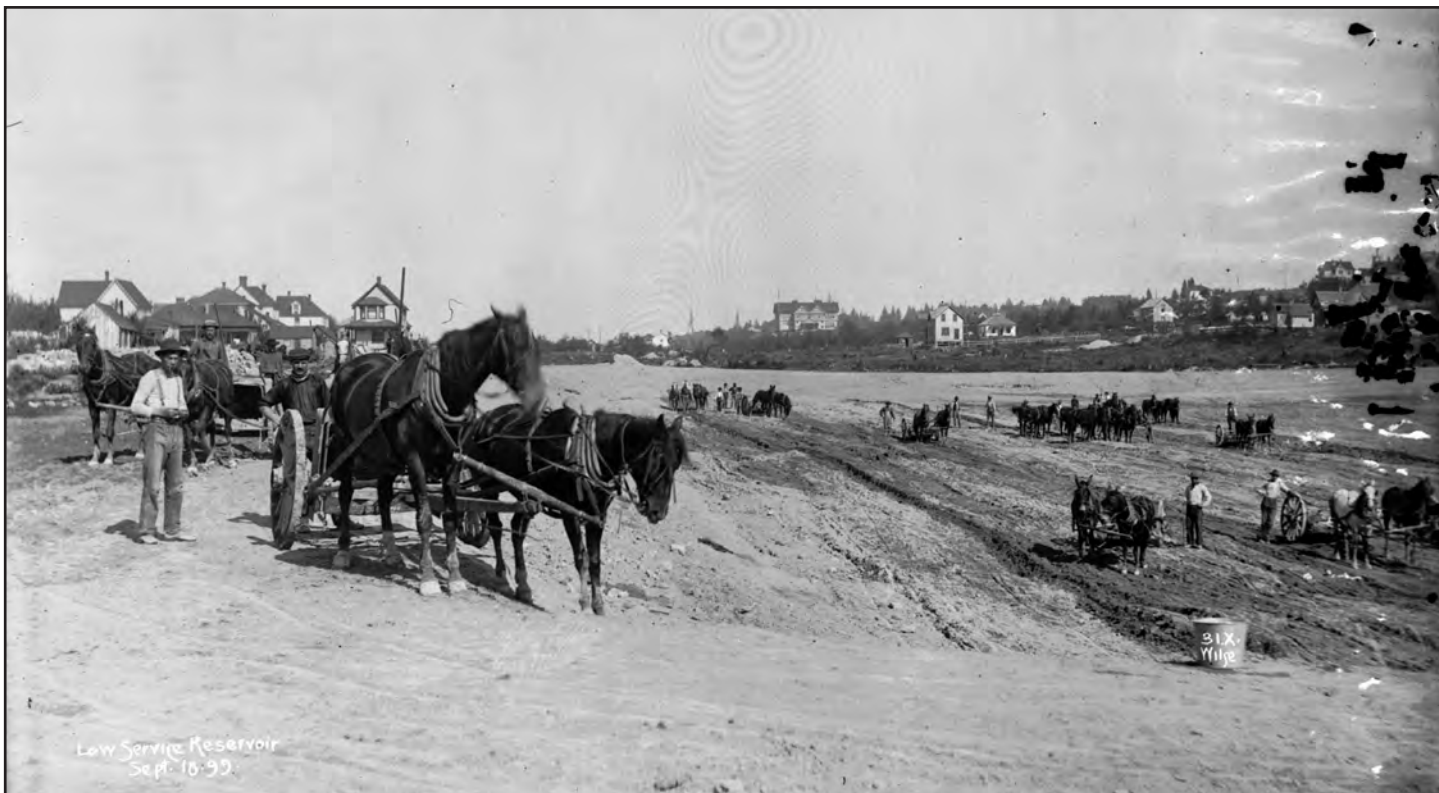
Figure 55 • Lincoln Reservoir under construction, September, 18, 1899
