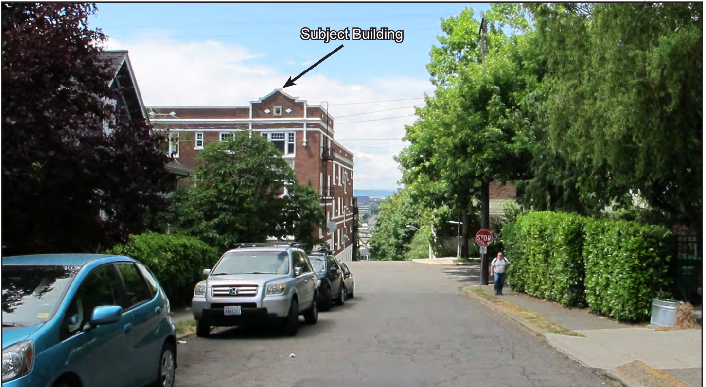
Figure 8 • View E - Viewing west on E Roy Street
