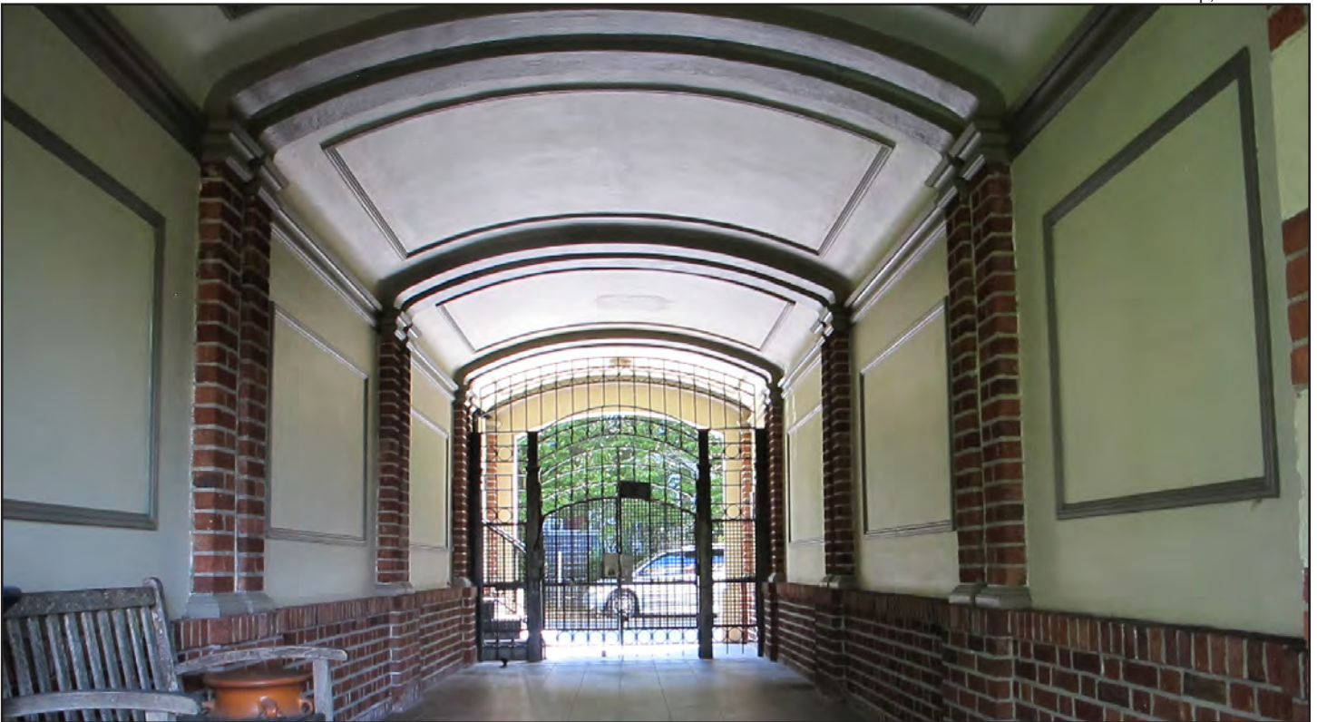
Figure 38 • Courtyard-east façade, entry corridor looking towards Bellevue Avenue E
