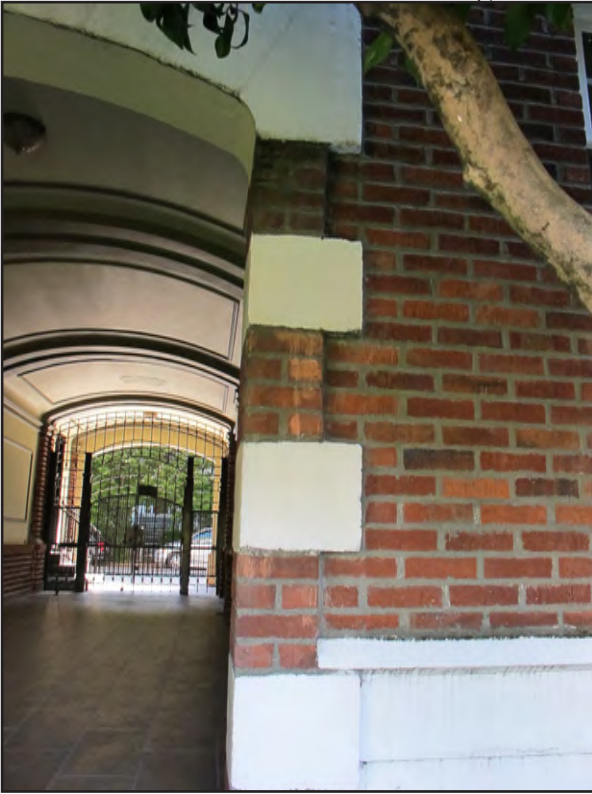
Figure 39 • Courtyard-east façade entry detail, painted cast-stone quoins
