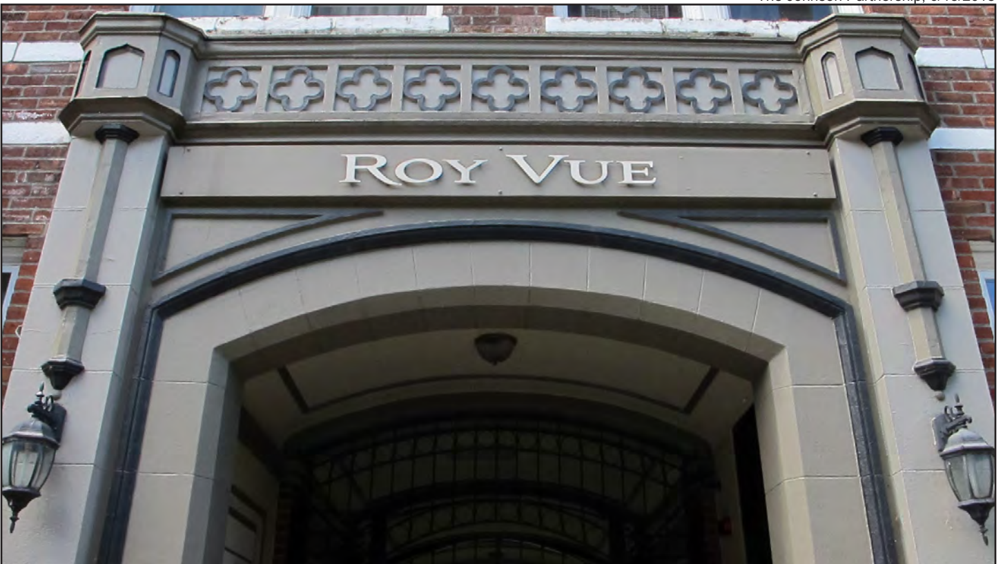
Figure 17 • Eastern façade, entry archway
