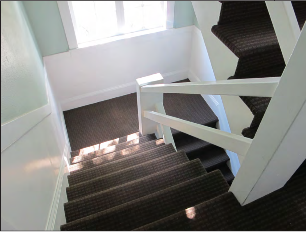
Figure 50 • Exterior stairwell, secondary vertical circulation from exterior entrance
