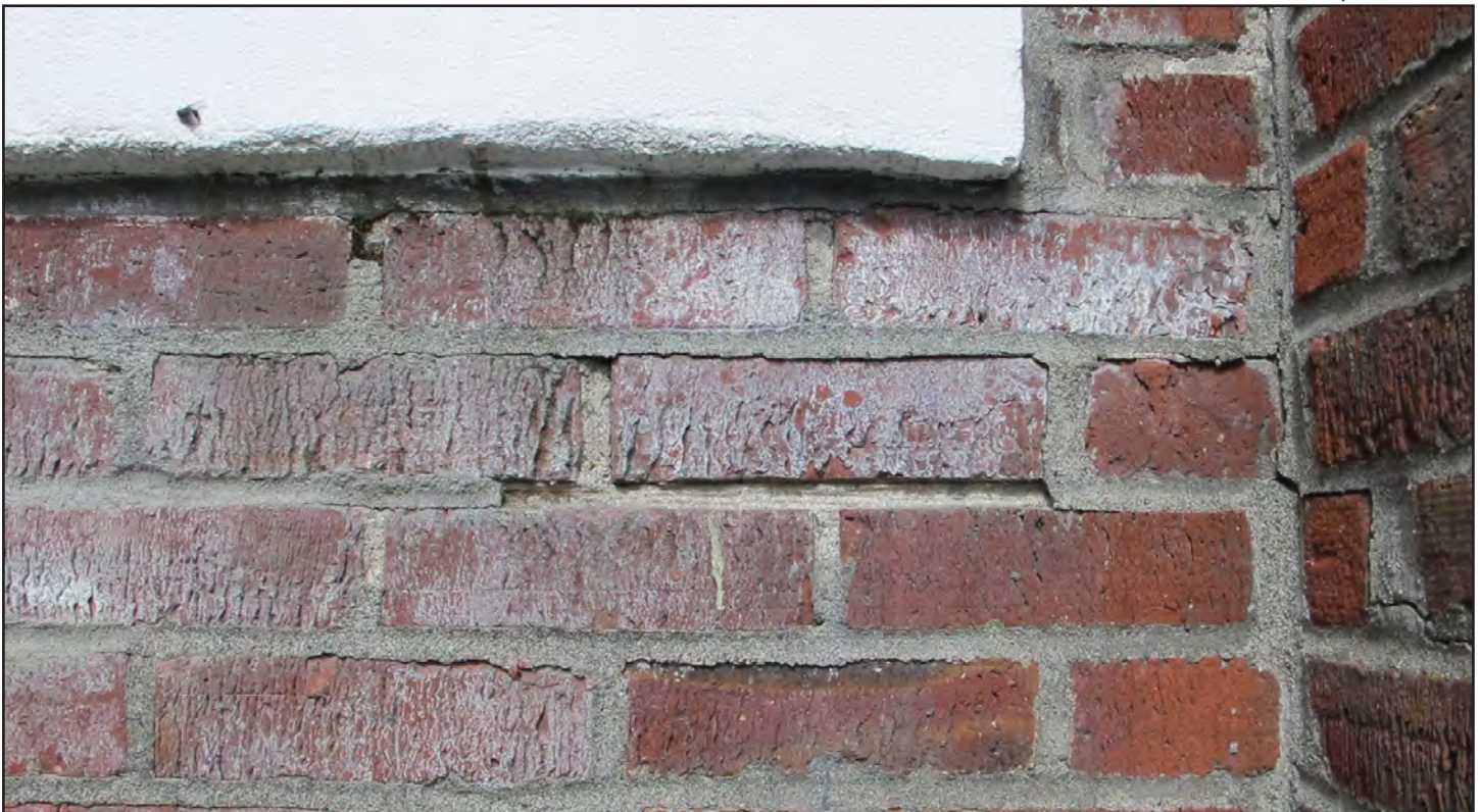
Figure 21 • Eastern façade, detail of cast-stone sill and brickwork
