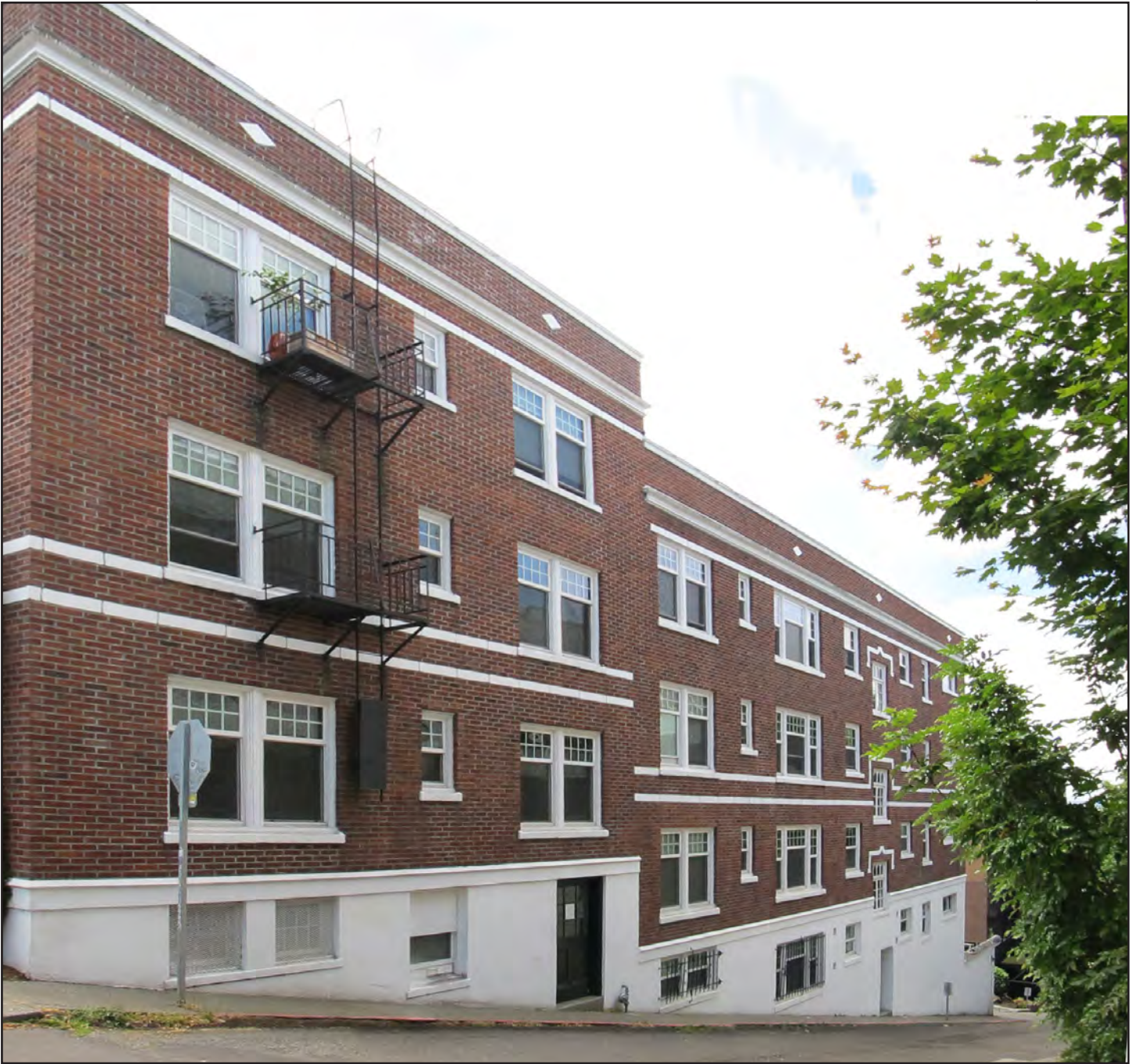
Figure 26 • Northern façade along E Roy Street
