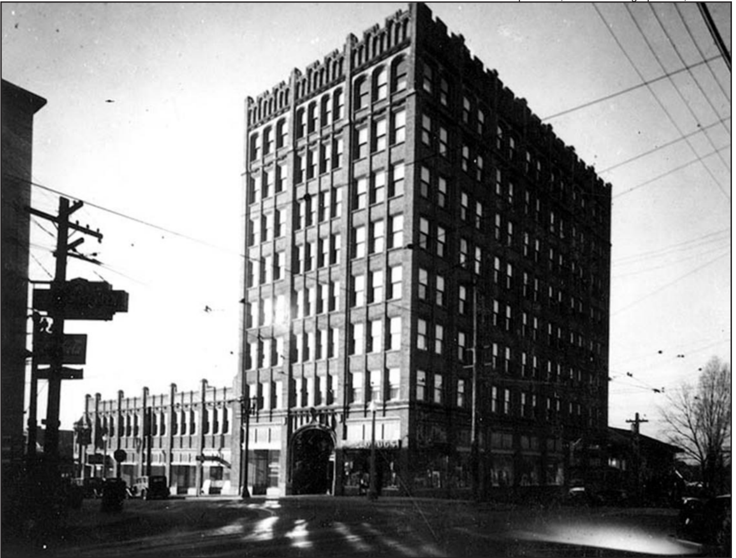
Figure 85 • Brooklyn Building (Brooklyn Avenue and N.E. 45th Street) circa 1929, built 1929.
