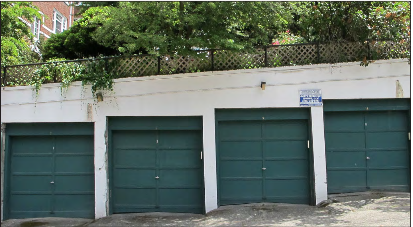
Figure 31 • Western façade, garage detail
