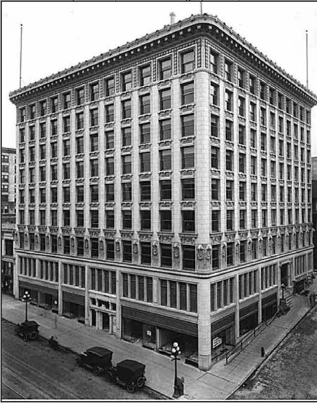
Figure 93 • Arctic Building (Warren Gould, 700 Third Avenue, City of Seattle Landmark), built 1917
