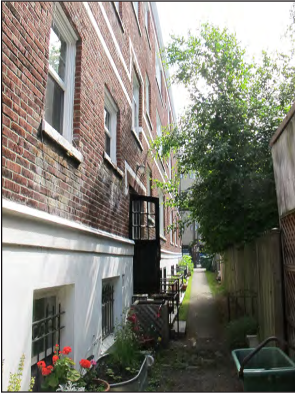
Figure 23 • Southern façade looking east
